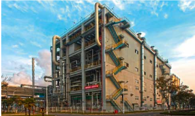
100 KT/A POLYCARBONATE POLYCONDENSATION PLANT
